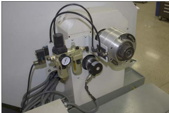
Figure 1-19: Air connections from the pneumatic cylinder to the solenoid.
