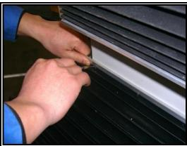
4. Using the 3.3mm drill bit and a small hand electric drill (if the electric drill is too big it will interfere with other parts while drilling) and drill the three holes at the scribed positions. See the photo on the next page.
